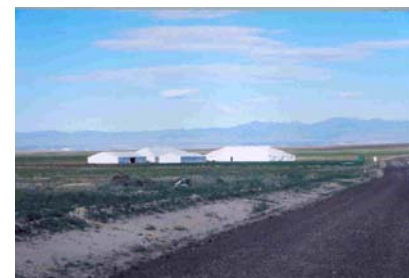
Temporary Barracks Gowen Field Training Center, ID
