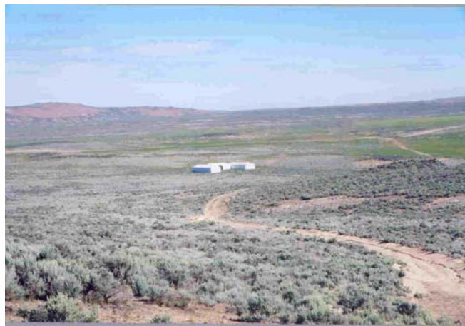
Remote Forward Operating Base Gowen Field Training Center, ID
